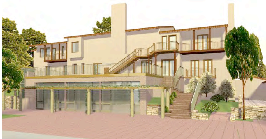
A new main entrance to the "back" of Founder's Hall. Stairs and an elevator lift allow access from the Chapel parking lot and Giesy Hall. An extension of the back deck creates a roof for the new Community Room.
