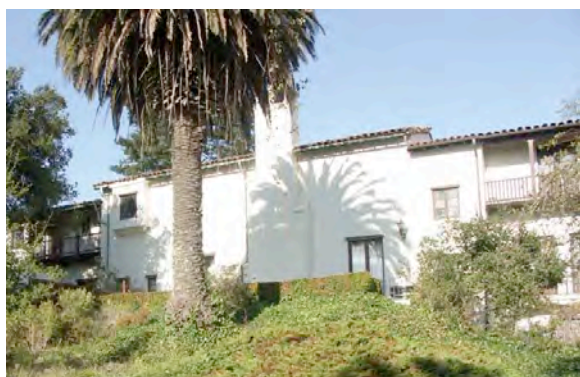
Photographs of the "back" of Founder's Hall. New exterior stairs to upper floor can wrap around chimney without blocking any existing windows. Existing stair hall will become new entry hall.
