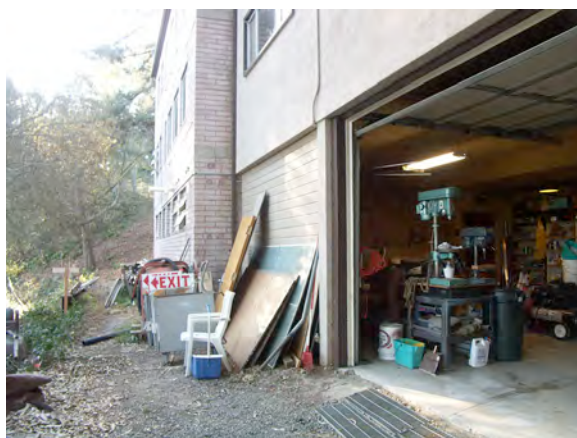
Current maintenance shop in the basement of Beasom could become a 4-BR apartment.
