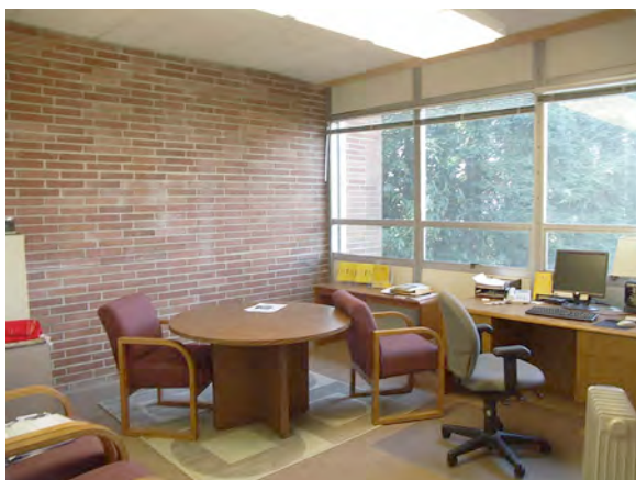
Solid brick structural walls are attractive where exposed on the interior.
